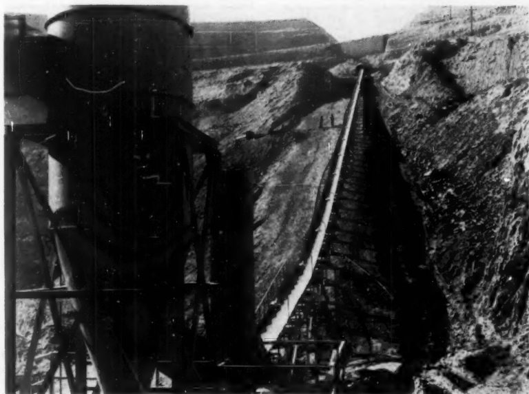
BELT is 1,300 feet long up 18° slope out of pit. Tunnel at top is midway point on belt. Cyclone at left is part of dust collecting system at crusher.
